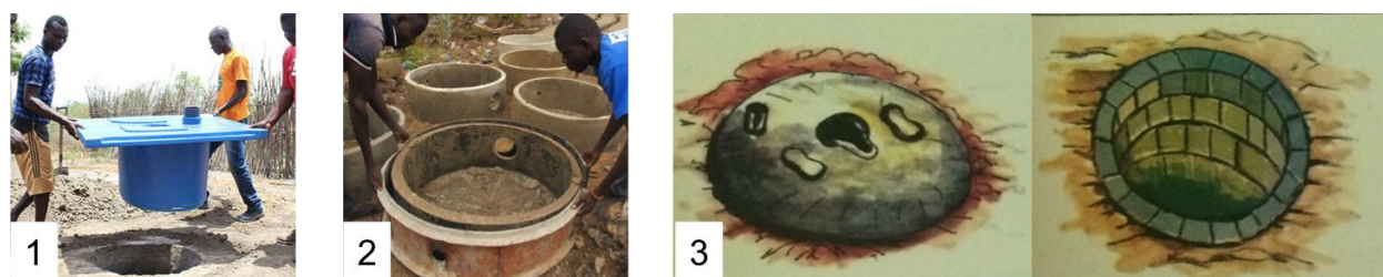
Figure 1: latrine options offered in the subsidy intervention: 1) Digni-Loo, 2) pre-cast concrete rings and slab, 3) Mozambique slab and masonry pit lining.
