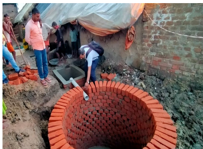
Figure 5. Construction of a Soak Pit in Bihar
