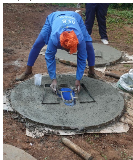
Woman installing SATO Pan (Picture Credit: PSJ)
