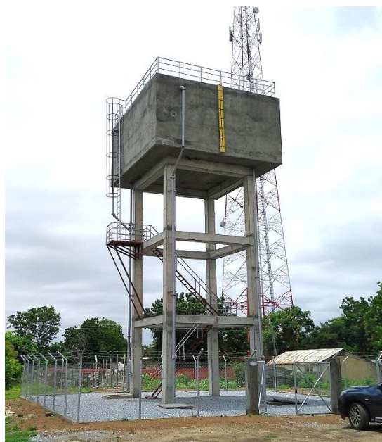
Photo 3: Water tank in the Tuna system
