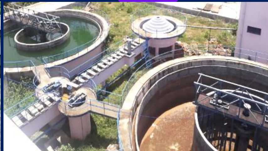
Water Supply Scheme, Bhubaneshwar, Odisha
