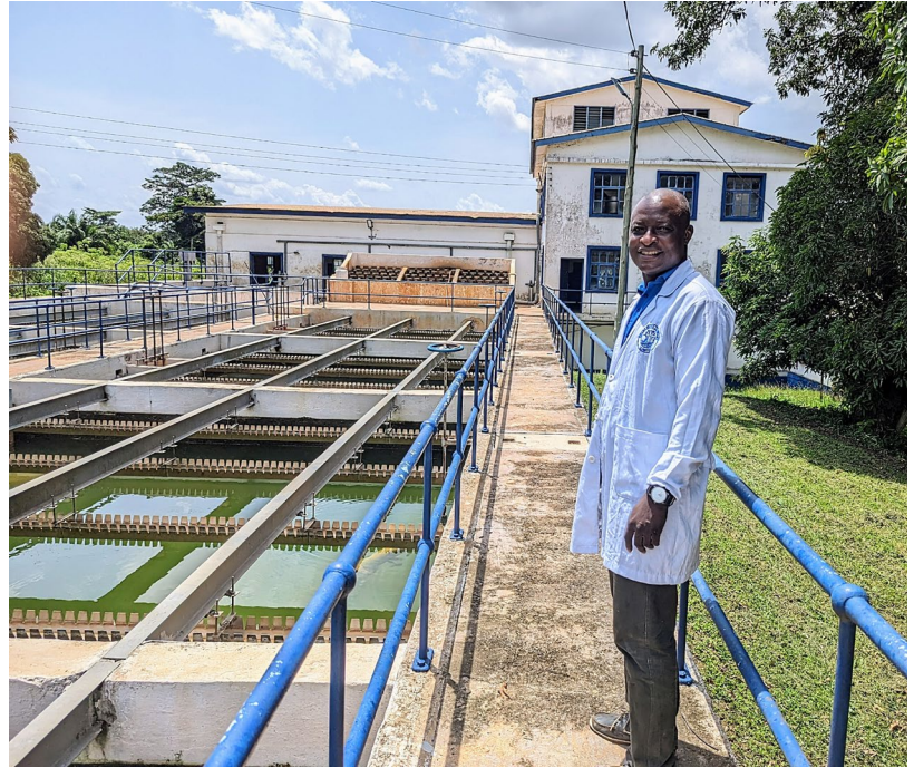
GWCL staff lead site visit of the Owabi water treatment plant in Ashanti region (sedimentation tanks pictured here).
