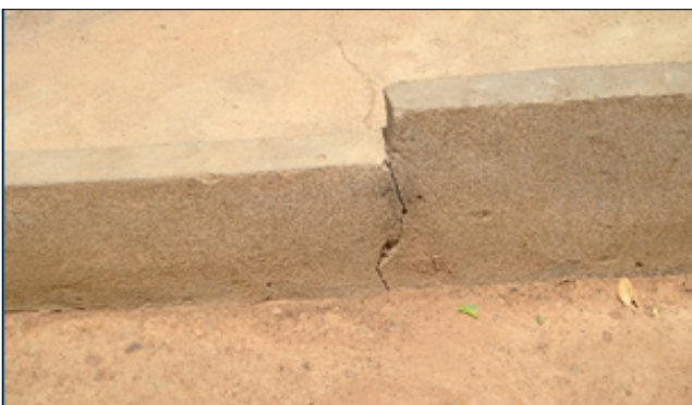
Does the water point have cement walls? Are there any cracks in the walls?
