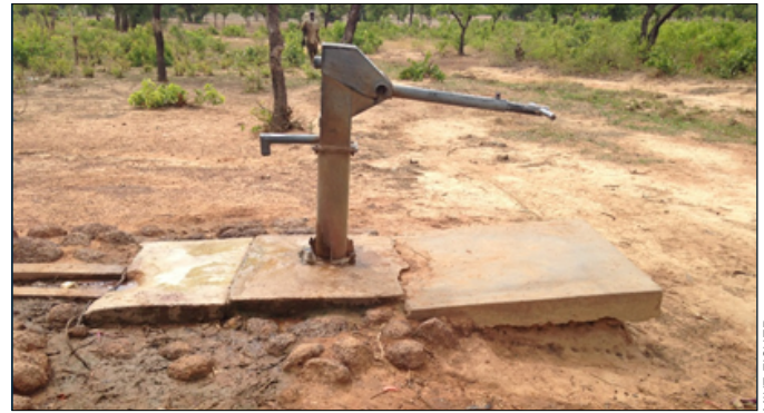
Does the water point have a full cement apron?
