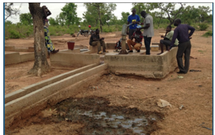
Does the water point have a cement floor? Is there any ponding of still water within 2 m of the floor?
