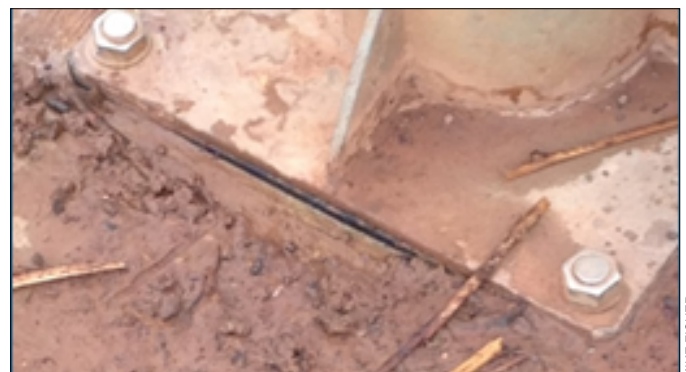
Is the base of the water point adequately sealed so that outside water can't enter?
