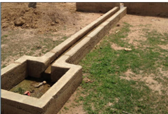
Does the water point have a drainage channel? Is the drainage channel broken, cracked or in need of cleaning? Is it full of still water?
