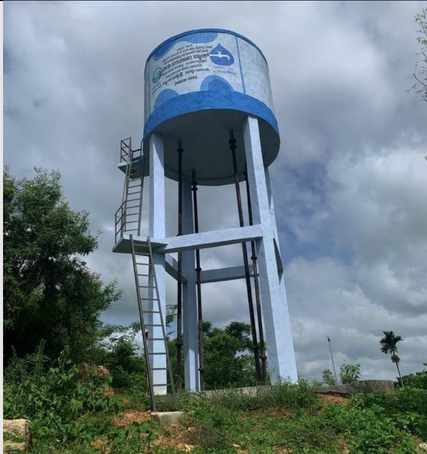
Figure A-3: Overhead tank at Lakshmipura village, Ramanagara district
