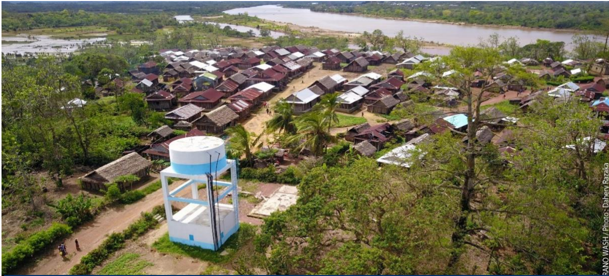
Picture 4. This new water tank built in Vohitrindry, Fitovinany region, has a capacity of 50m 3 , and allow over 10,000 people to drink
