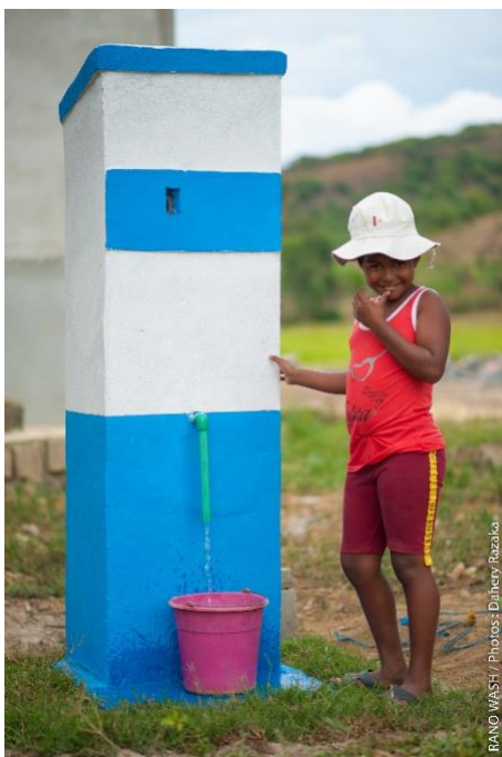
Automatic water kiosk in Alaotra Mangoro Region
