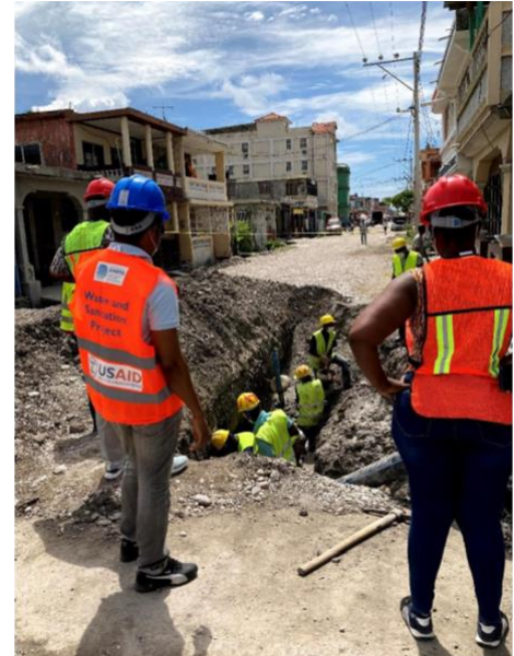
Repairing water pipes in Les Cayes. Credit: DAI Global for USAID (2021)
