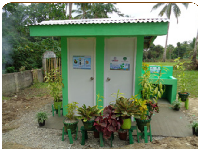
Gender segregated twin cubicle toilet with handwashing facility at Sto Nino school in Leyte
