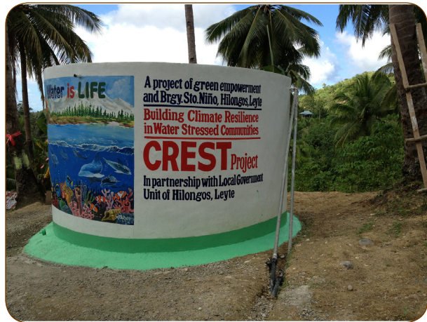
A completed water tank in Brgy. Sto. Niño, Hilongos, Leyte, after the community has decorated it.
