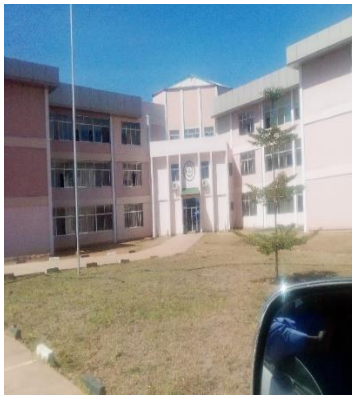
FIGURE 15. CHINSALI COUNCIL OFFICES-BACK VIEW
