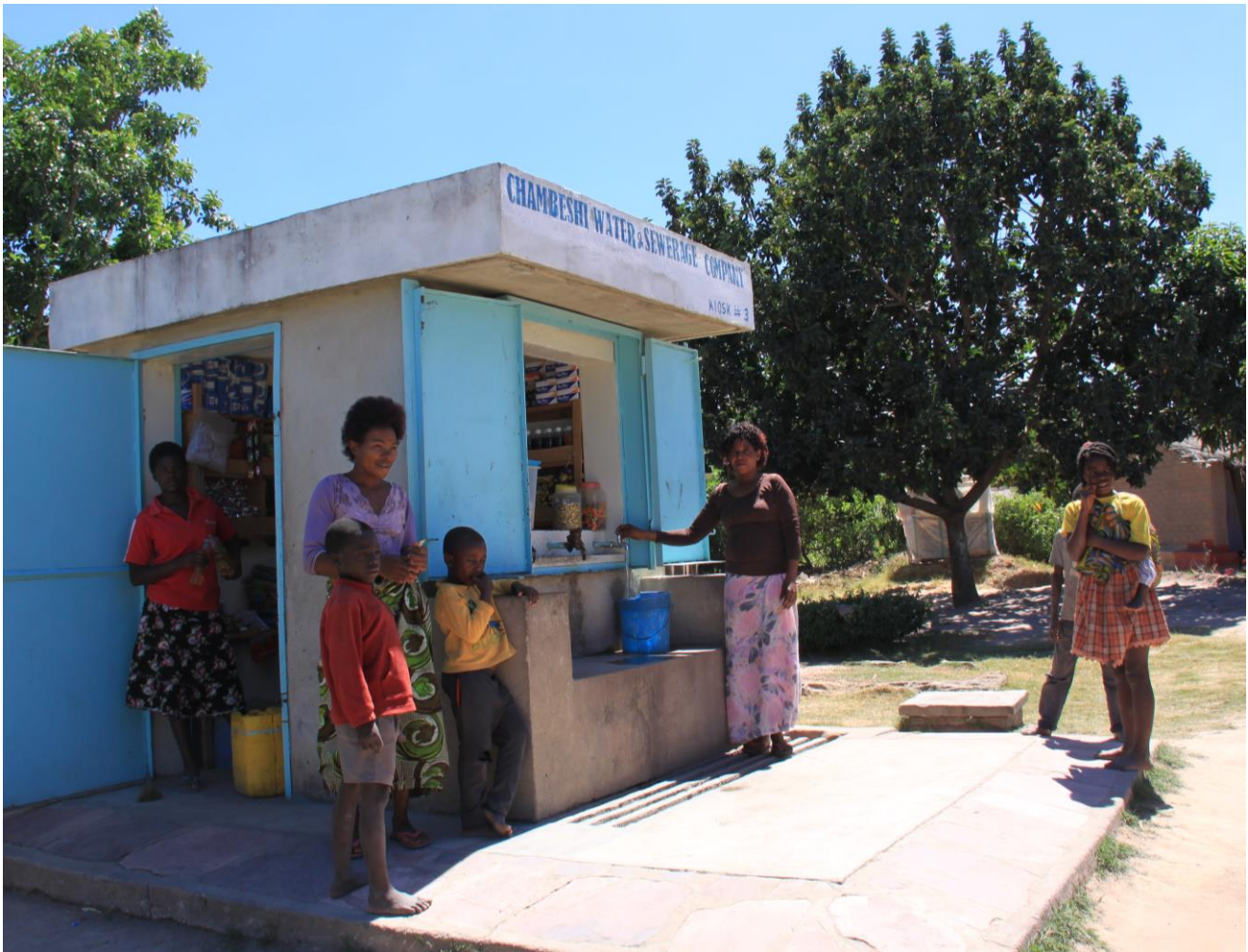
PHOTO CAPTION: Water kiosk operated by Chambeshi Water and Sewerage
