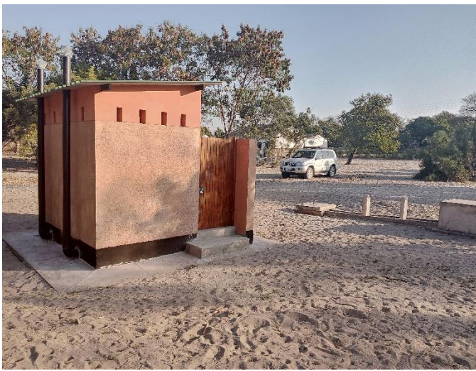
A. A completed toilet with an incomplete washing facility in front
