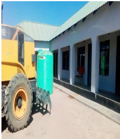
FIGURE 23. LUNTE COUNCIL OFFICES
