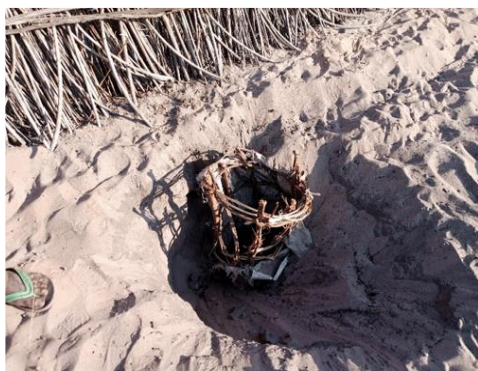
FIGURE 8. POORLY CONSTRUCTED SUBSTRUCTURE
