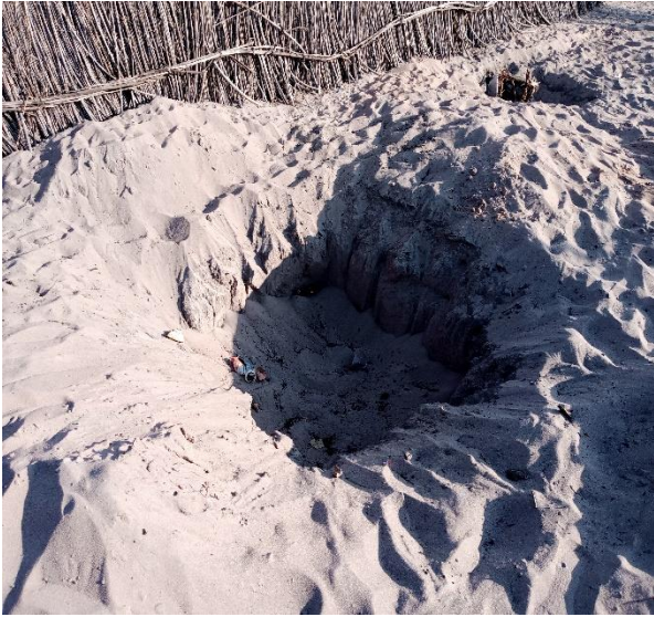
A. Poorly Excavated Refuse pit
