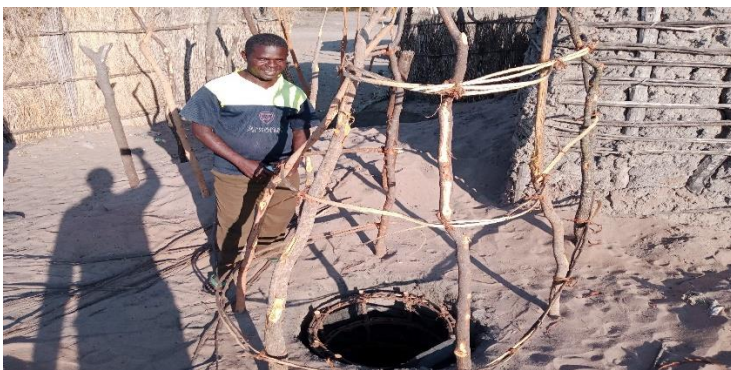
C. Community Sanitation Champion demonstrating how to frame the toilet super structure
