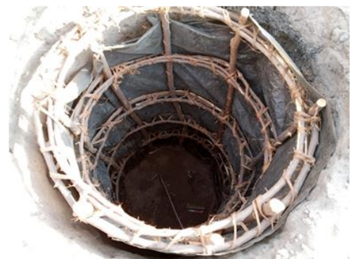
FIGURE 9. A WELL-PLACED TOILET RING IN MUYONGO VILLAGE IN KAMA
