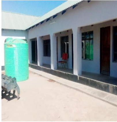
FIGURE 20. LUNTE COUNCIL OFFICES
