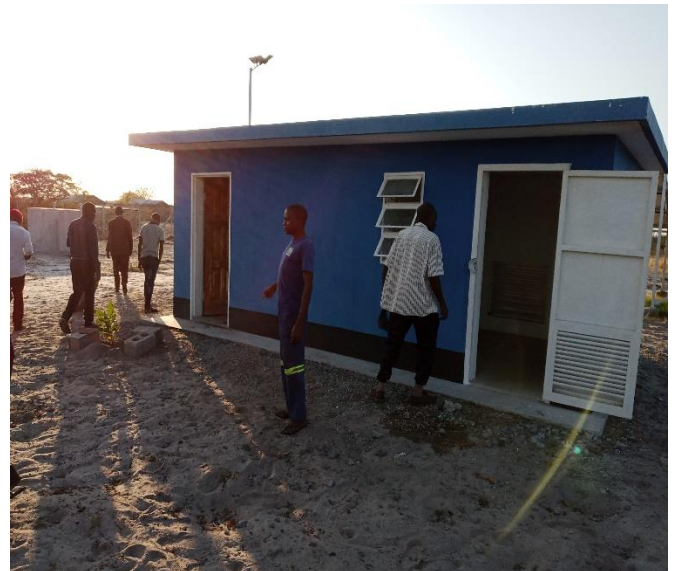
D. The Pump House for Kama Water Scheme.
