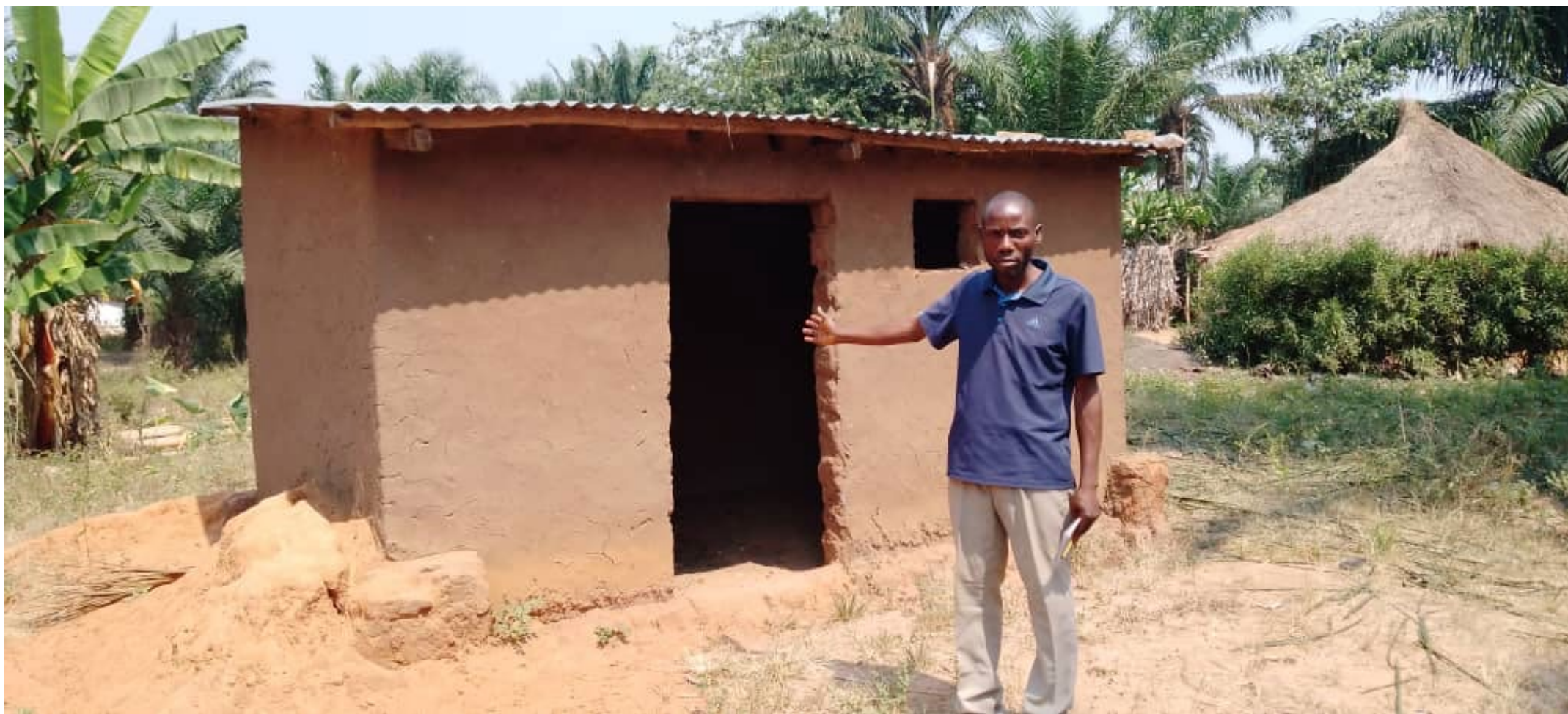
The newly built pharmacy building from the Tshilamba committee's IGA.
