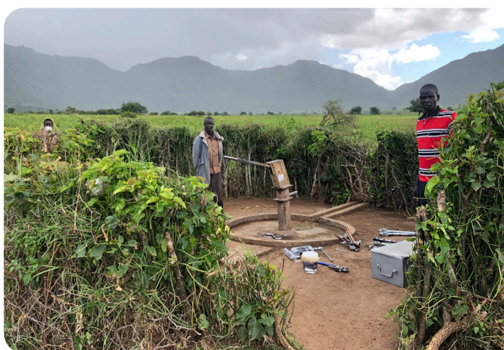
Water point near Karenga undergoing maintenance.
